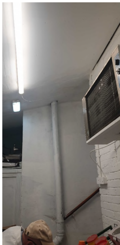
Dirty walls in dry store area
