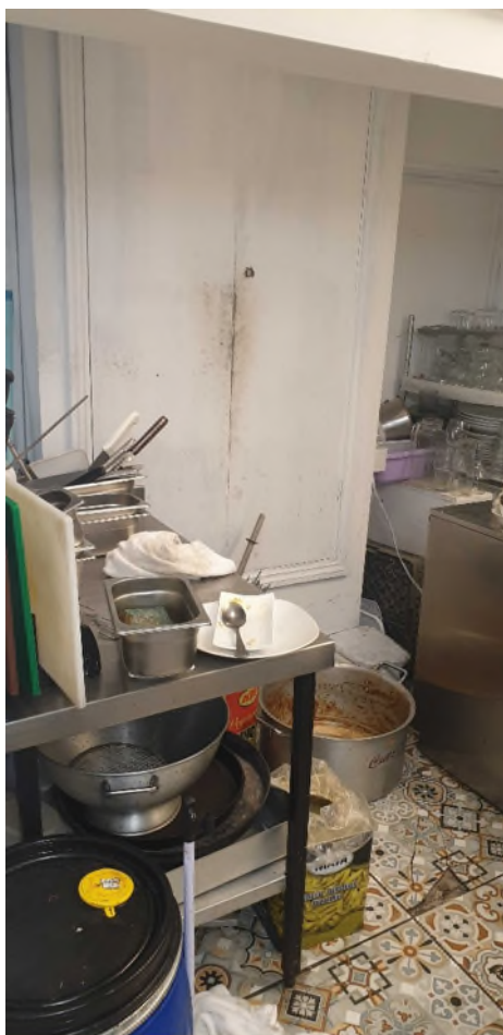
Dirty cupboard doors and broken tile upper rear preparation room
