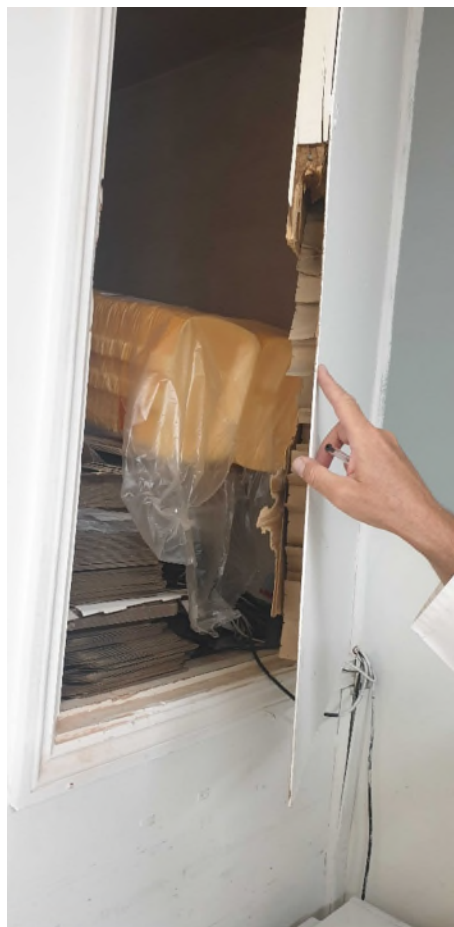
Bare hardboard exposed in cupboard in upper rear preparation room
