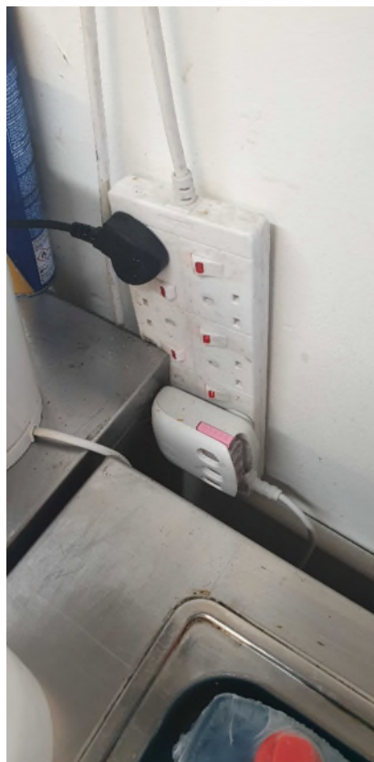
Dirty electric socket points in rear upper kitchen
