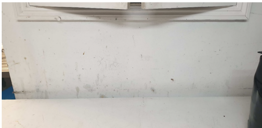
Wall stained in upper rear preparation room
