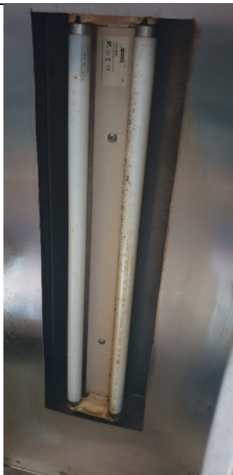
Staining and no diffusers to lights in canopy
