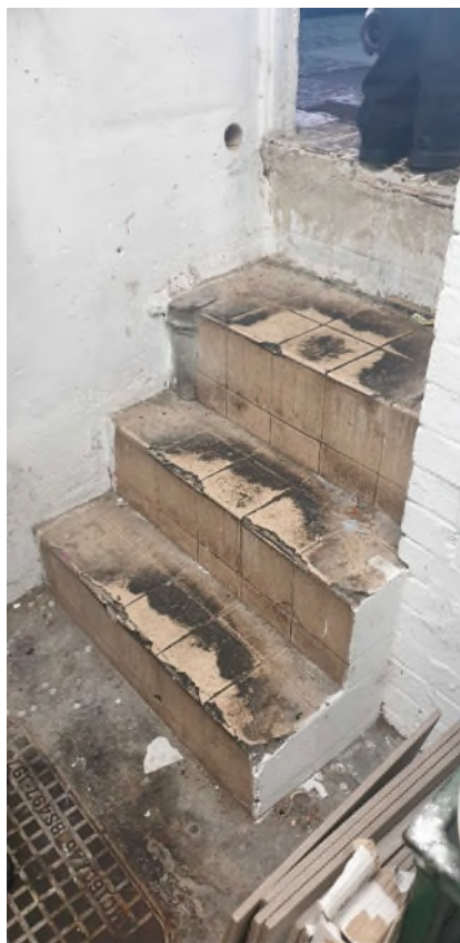
Damaged floor tiles on steps from dry store
