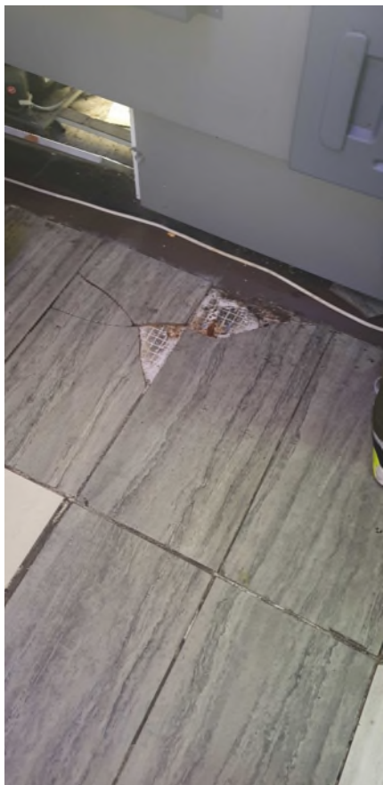
Broken floor tiles to rear of display fridge in serving area
