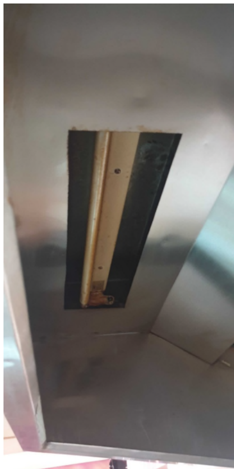
Staining and no diffusers to lights in extract canopy
