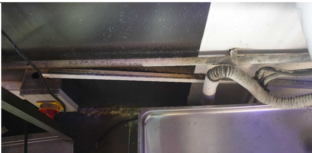
Debris and dirt accumulation to rear of display fridge
