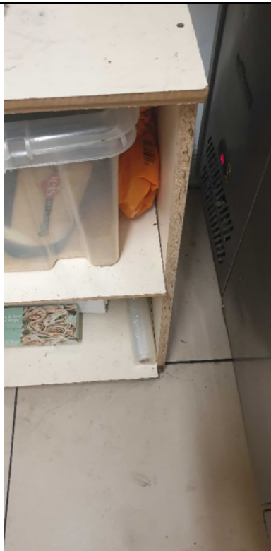
Bare chipboard exposed in cabinet rear upper preparation room
